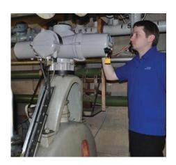
new IQ3M actuators that are specifically designed for modulating duties. Because there is a constant demand to use the wind tunnel, the retrofit operations can completed in the brief periods available between test programmes. The first two actuators were removed and the replacement IQ3M actuators installed and commissioned in two days, half the allocated time allowed before the wind tunnel was due to re-start operations.
