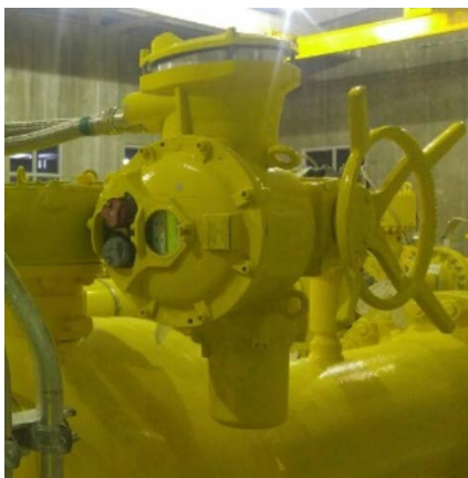
Bernard Controls' explosionproof actuators (yellow paint specification on customer request)
