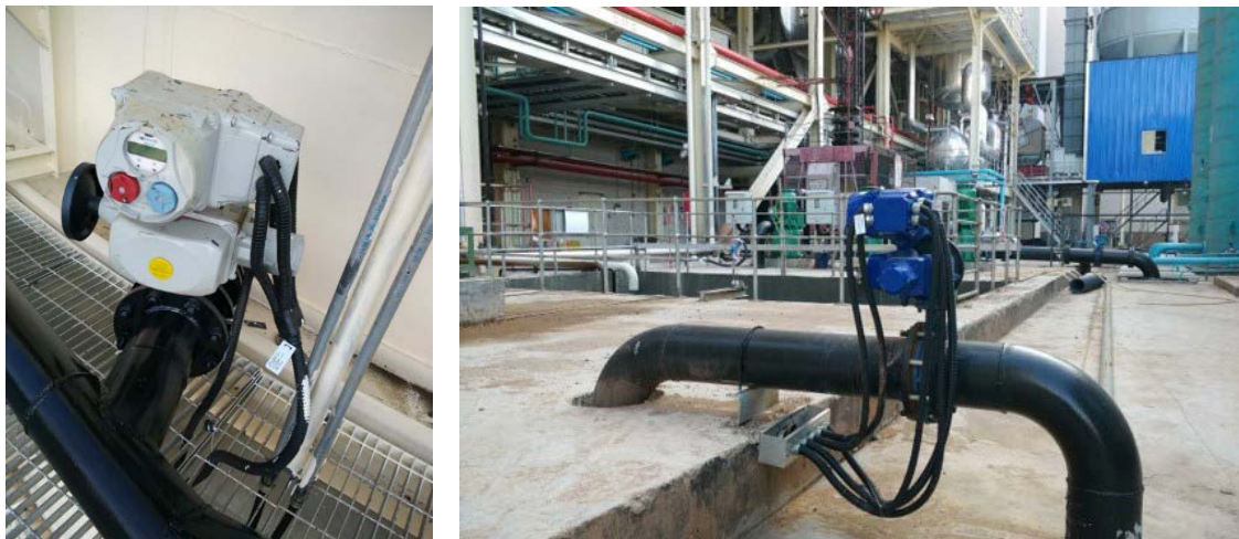
Bernard Controls' quarter-turn SQ actuators mounted on valves on Dapu Thermal Plant
