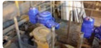
BERNARD CONTROLS' actuators used to motorize the dampers (+22m)
