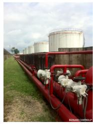
End of 2014, BERNARD CONTROLS delivered and setup more than 120 explosionproof quarter-turn actuators (SQX models) with INTELLI+® intelligent integrated control, to automate an oil depot fire protection located in Douala (Cameroon) for SCDP (Société Camerounaise des Dépôts Pétroliers).
